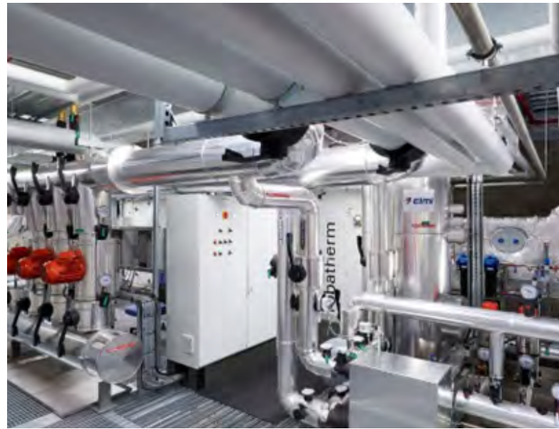
Installation ligne BFS – Recipharm Kaysersberg (68)
